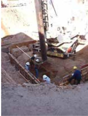
Setting casing for hydraulic cylinder.
