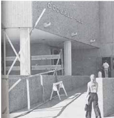
Photo from the 1977 yearbook. Photo shows the re-enforcing supports on the building while efforts were made to prevent the building from “sinking”.
