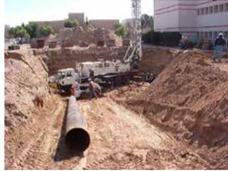
Drilling hole for elevator hydraulic cylinder.
